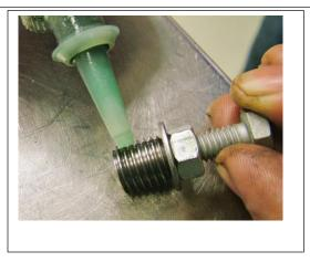
Step 14. Install the insert until the washer bottoms against the head. Back the nut on the installation toll away from the washer while holding the bolt securely.
